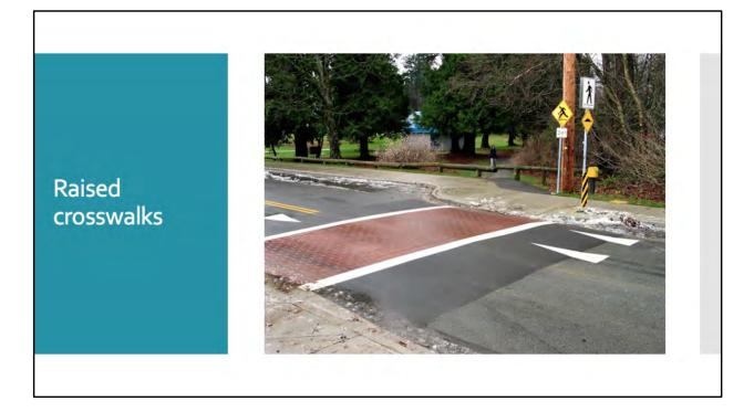
Raised crosswalk combines a speed hump and a crosswalk (red colouring in this example is an optional extra treatment) Can reduce 85th percentile traffic speeds by 5 to 13 km/h Also increase proportion of motorists who yield to pedestrians (example from Delta)
